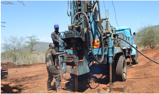
Borehole sinking in Kajiado to combat drought.
