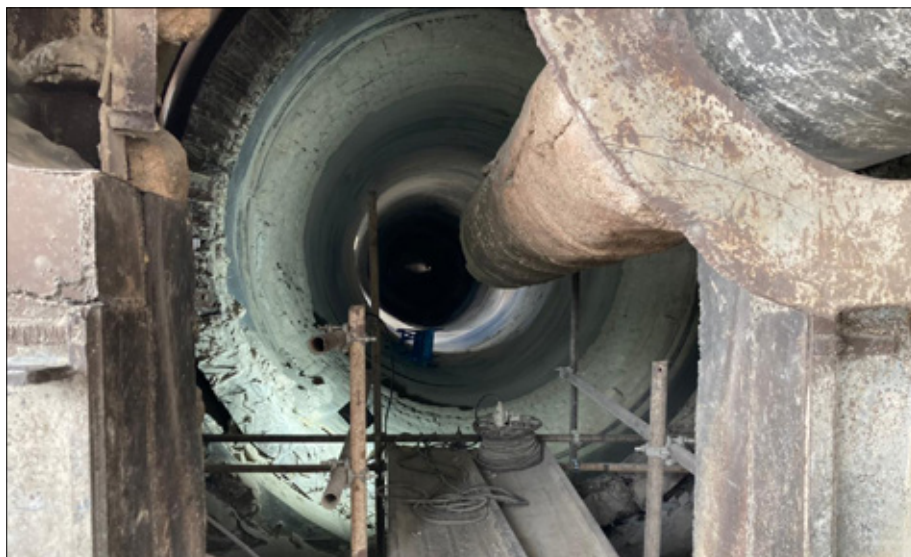
De-bricking of the inner kiln shell.
