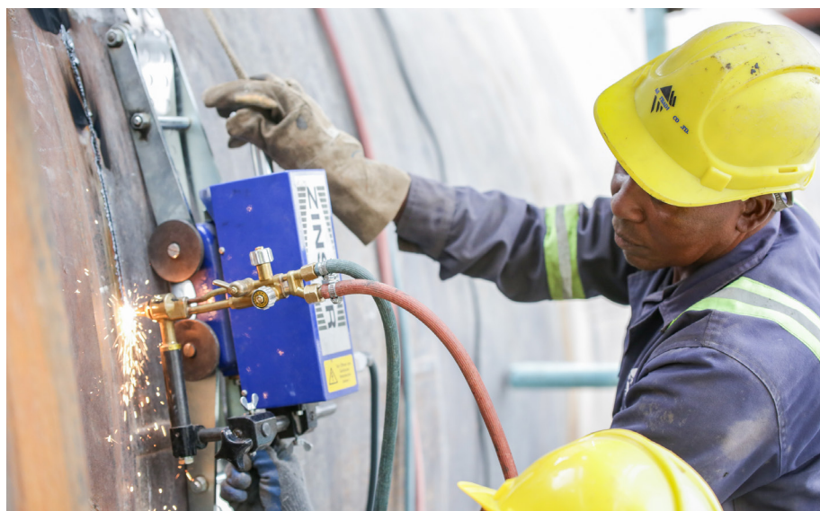
Ongoing works on the kiln shell.
