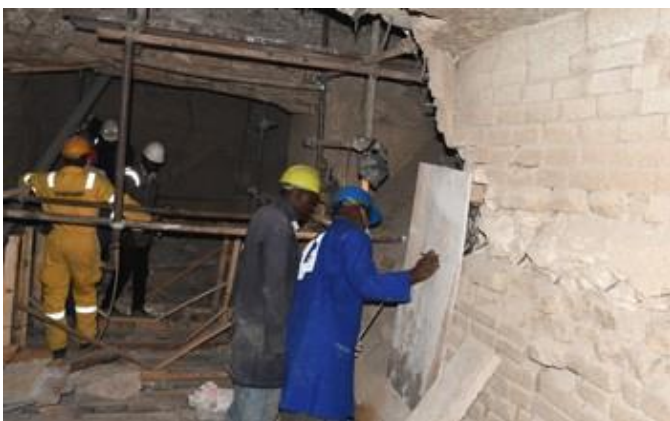
Final works ongoing in the grate cooler.
