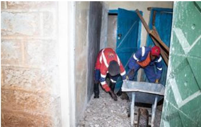
Construction workers embark on the rehabilitation works after receiving the cement.
