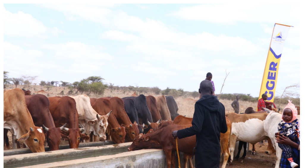
Community livestock drink from a Water Trough connected to the Borehole
