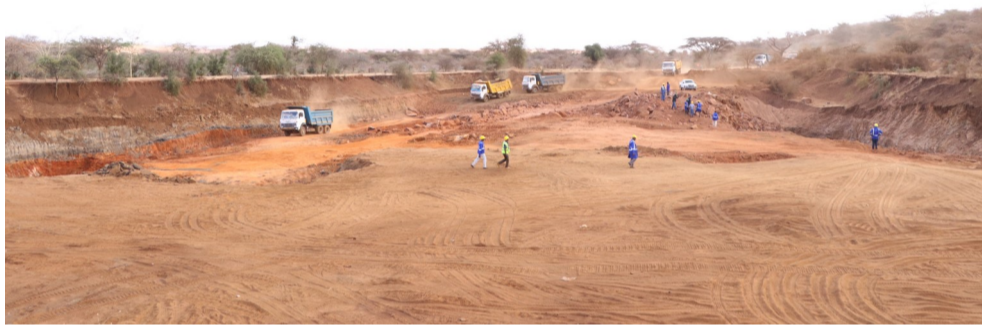
Trucks drive back into the Pit after the blasting
