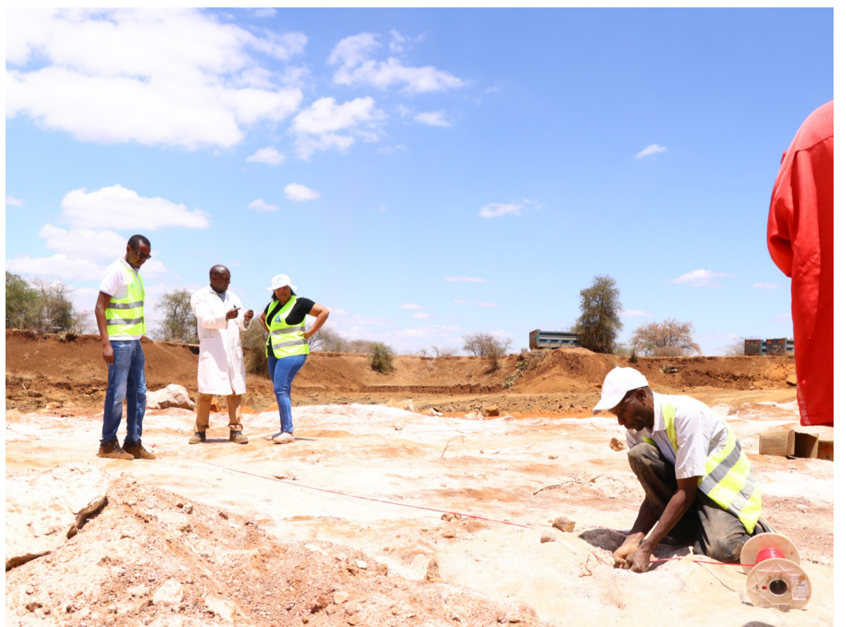
Setting up of explosives for the blasting in progress
